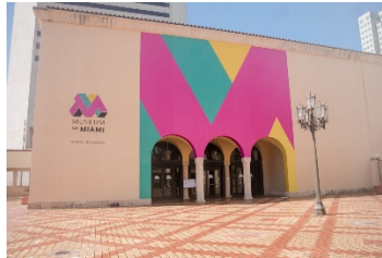
Above: The Museum of Miami- Entrance to the North Building 101 West Flager Street, Miami, Florida 33130
